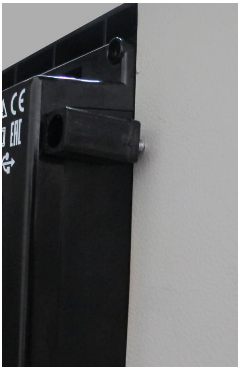
Installation of screw type bracket
